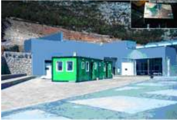
Prefabricated Technology (Raymond, 2001)
