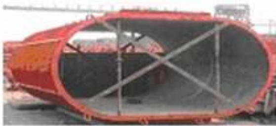
Tunnel formwork (Raymond, 2001)
